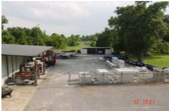
Yard View Of MCLA Shop
